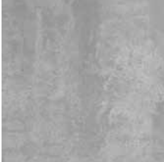
Concrete hell (DP*)
