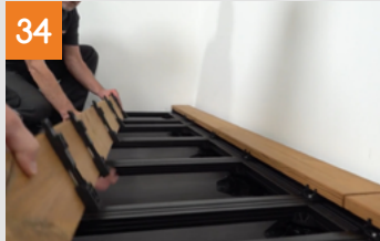
Installation of the boards over an area
