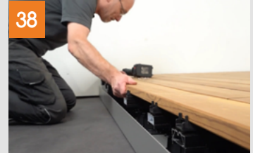
Installation of the last board
