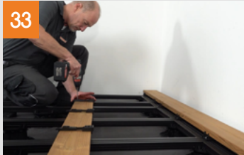
Installation of the boards over an area
