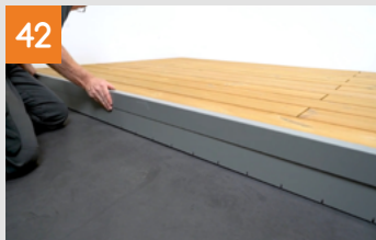
Completion of the side panel
